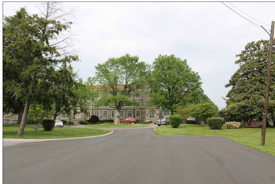
VIEW OF ST. PAUL'S COLLEGE (1913 WING) AND CIRCLE FROM EXISTING PARKING LOT
